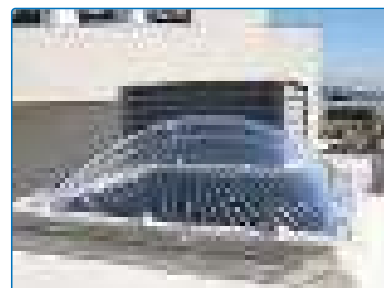
Bivalve skylight with protection net
